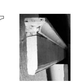
SALVAGED WINDOW HEAD TRIM PROFILE, SAND/REFINISH WITH FIELD STAIN, <u>OR</u> PROVIDE NEW 4" X 3/4" WHITE OAK TRIM WITH SAME PROFILE, FIELD STAIN, MITERED CORNERS FOR FINISHED RETURN TO WALL
