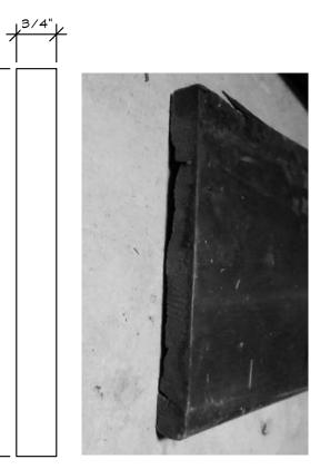
SALVAGED WOOD BASE PROFILE, SAND/REFINISH WITH FIELD STAIN, <u>OR</u> PROVIDE NEW 7 1/4" X 3/4" WHITE OAK TRIM WITH SAME PROFILE, FIELD STAIN, MITERED CORNERS FOR FINISHED RETURN TO WALL.
