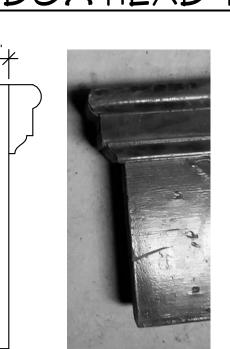
SALVAGED WINDOW HEAD TRIM PROFILE, SAND/REFINISH WITH FIELD STAIN <u>AND/OR</u> PROVIDE NEW 5-1/2" X 1-1/8" WHITE OAK TRIM WITH SAME PROFILE, FIELD STAIN, MITERED CORNERS FOR FINISHED RETURN TO WALL SALVAGED (AND/OR NEW WHITE OAK) VERTICAL TRIM TO BE 4 3/8" X 3/4" WITH SQUARE EASED EDGE, SAND/REFINISH WITH
